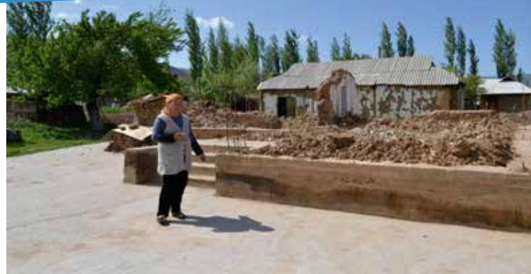
April 2016, Chaychi village, Osh oblast, Kyrgyzstan. Isakunova Svetlana talks about her destroyed house, which was damaged during the earthquake in 2015. (@OCHA / M. Sadvakasova)
